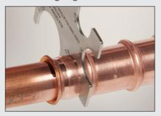
Verify the finished press band diameter by using the RLS press gauge. Find the proper size slot on the gauge and slide it over the press band. It should fit snug, but completely over the band. If not, the fitting must be re-pressed.
